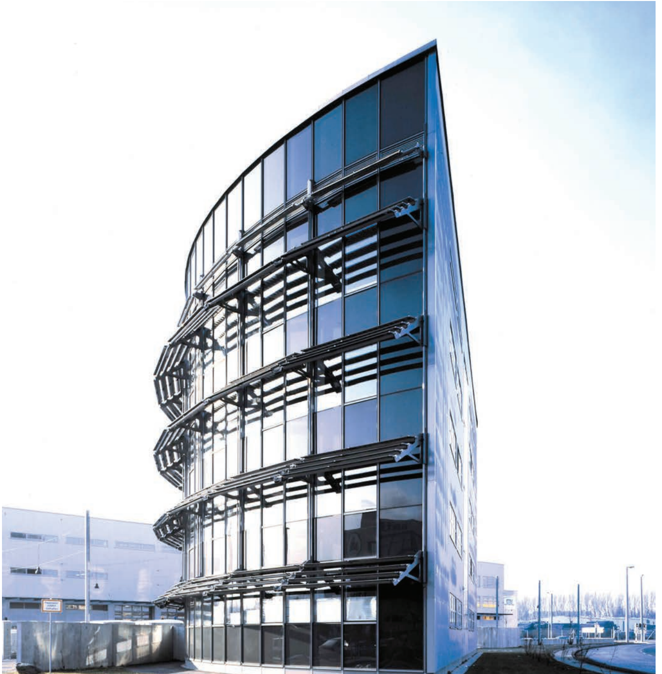
SBL Offices, Austria.
